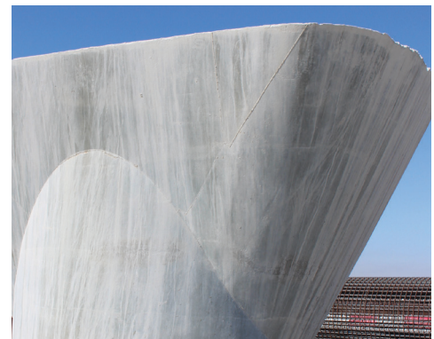
Formtex® withstands the challenges and ensures a strong and intact surface of the finished bridge pillar.
