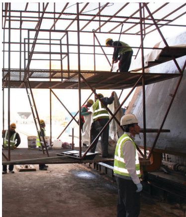
Formtex® is attached to the moulds with a special glue.
