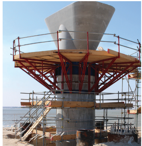
The tested and approved prototype of a bridge pillar.
