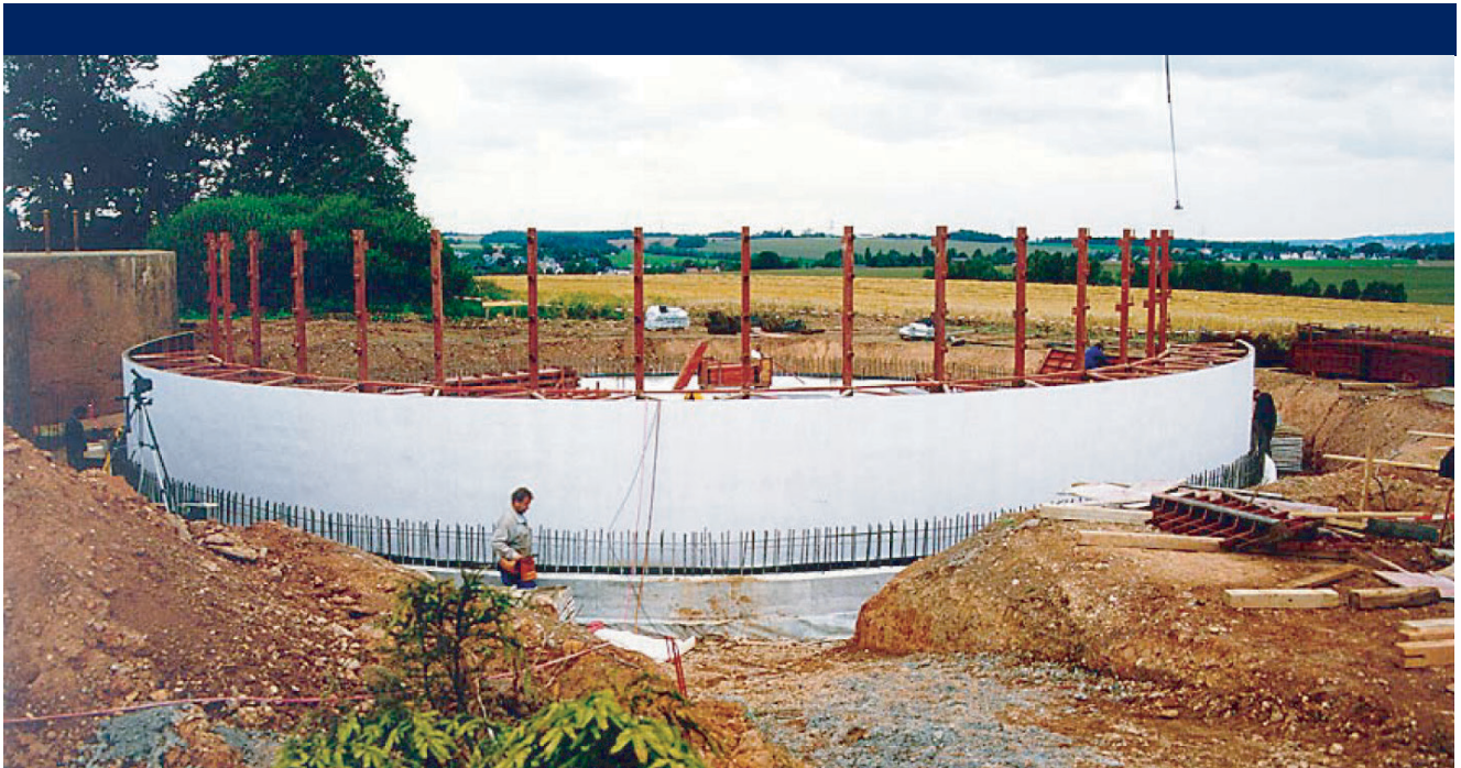
Figure 1. Drinking water tank before casting. The formwork elements have been lined with Formtex®.
