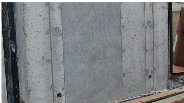
Figure 2. A trial for installation of Formtex® (middle).
