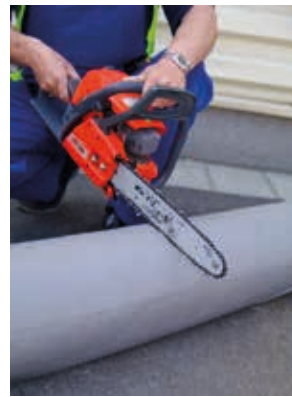
8.2 Cutting the Fibertex roll with a chainsaw
