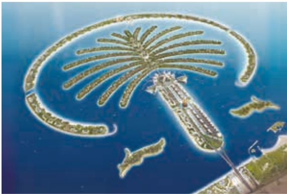
Figure 1.2 Fibertex Geotextiles were used in the Palm Islands
