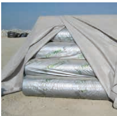
Figure 8.3 Correct storage on site
