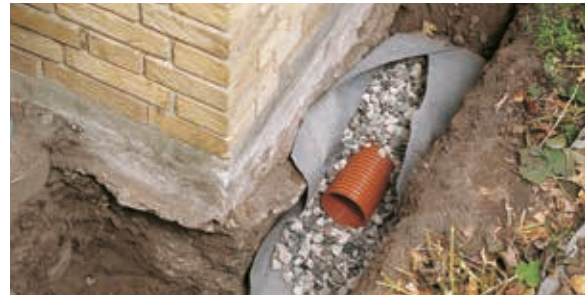
Figure 6.7 Example of a drainage trench installation
